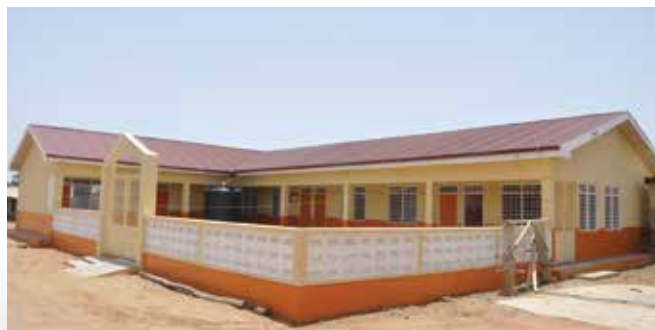
3-Unit Kindergarten Block at Korle-Gonno Cluster of Schools
