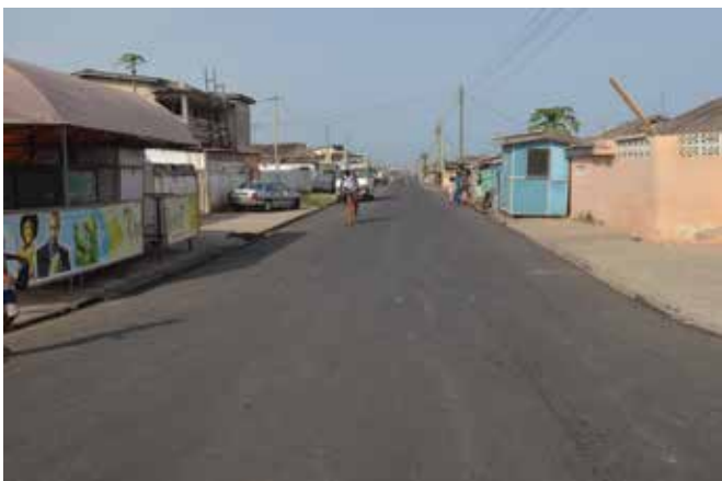
Asphalt Overlay within the Korle-Gonno Community
