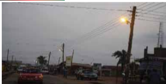
Installation of Streetlights at Chorkor
