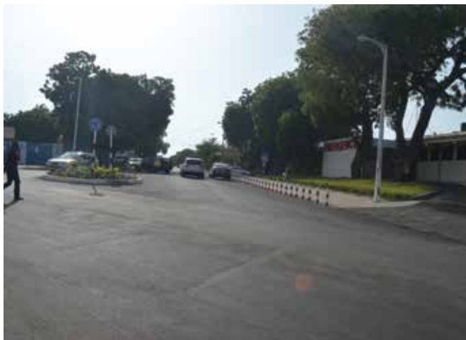
Asphalt Overlay at Korle-Bu Hospital
