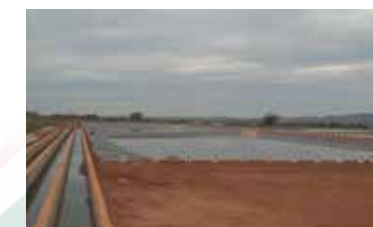
Completion of the Legon Treatment Plant
