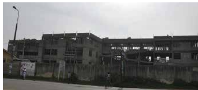
On-going Millennium City School at Korle-Gonno Cluster Of Schools
