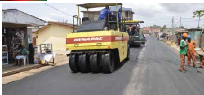
Asphalt overlay from Summer-hat to Banana-inn
