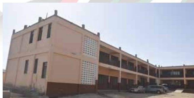
Construction of 2 Storey 12 Unit Class Room Block at Nanka Bruce, Korle Gonno
