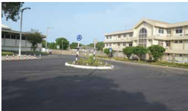
Asphalt Overlay at Korle-Bu Hospital
