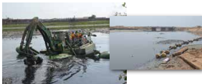
On-going Dredging of the Korle Lagoon
