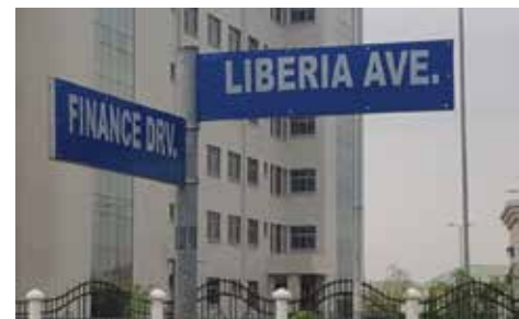
Installation of Street Signage within the City
