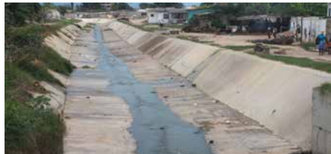
Mamponse Storm Water Drain
