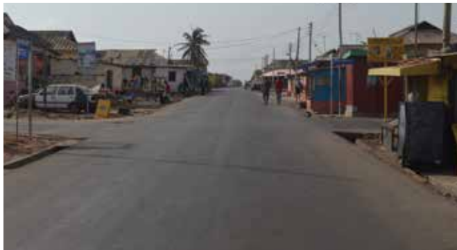
Asphalt Overlay within the Korle-Gonno Community
